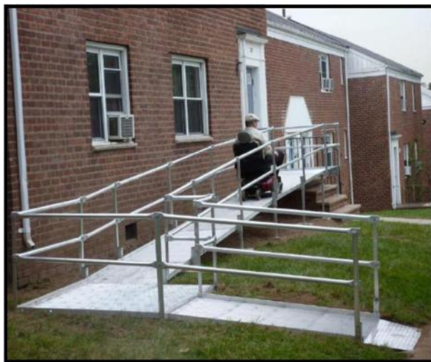
Accessible Ramp with Handrails for PwDs
