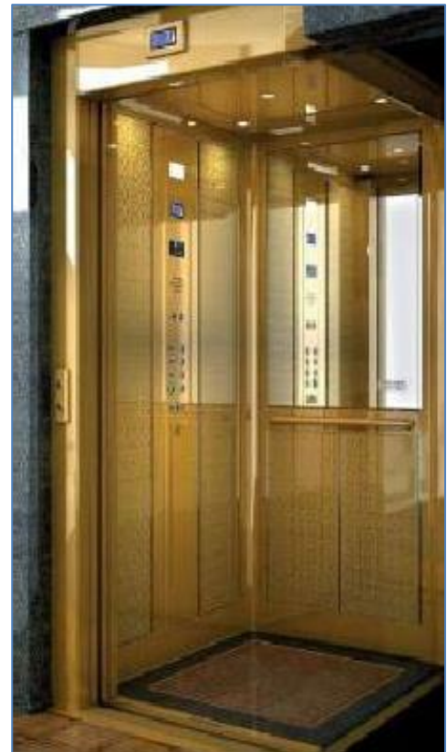
Accessible Elevator with Grab Bar, Mirror and auditory floor announcement system
