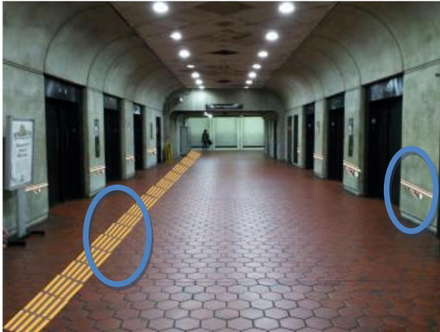
Accessible Corridors with Tactile flooring and low height grab bar as highlighted
